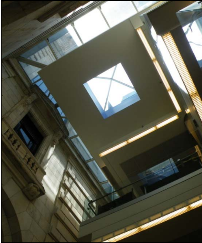
Figure 55: South Court Ceiling
